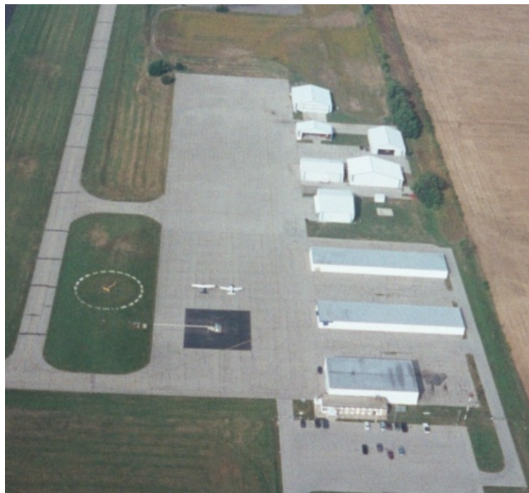
Picture 1: Aerial view of the terminal building, apron, vehicle parking & Hangars
